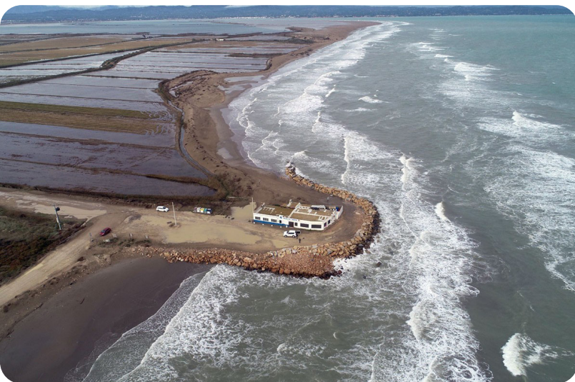
Rigid coastal structure protecting the Vascos restaurant. Photo: Taula de Consens, Aguaita.cat
