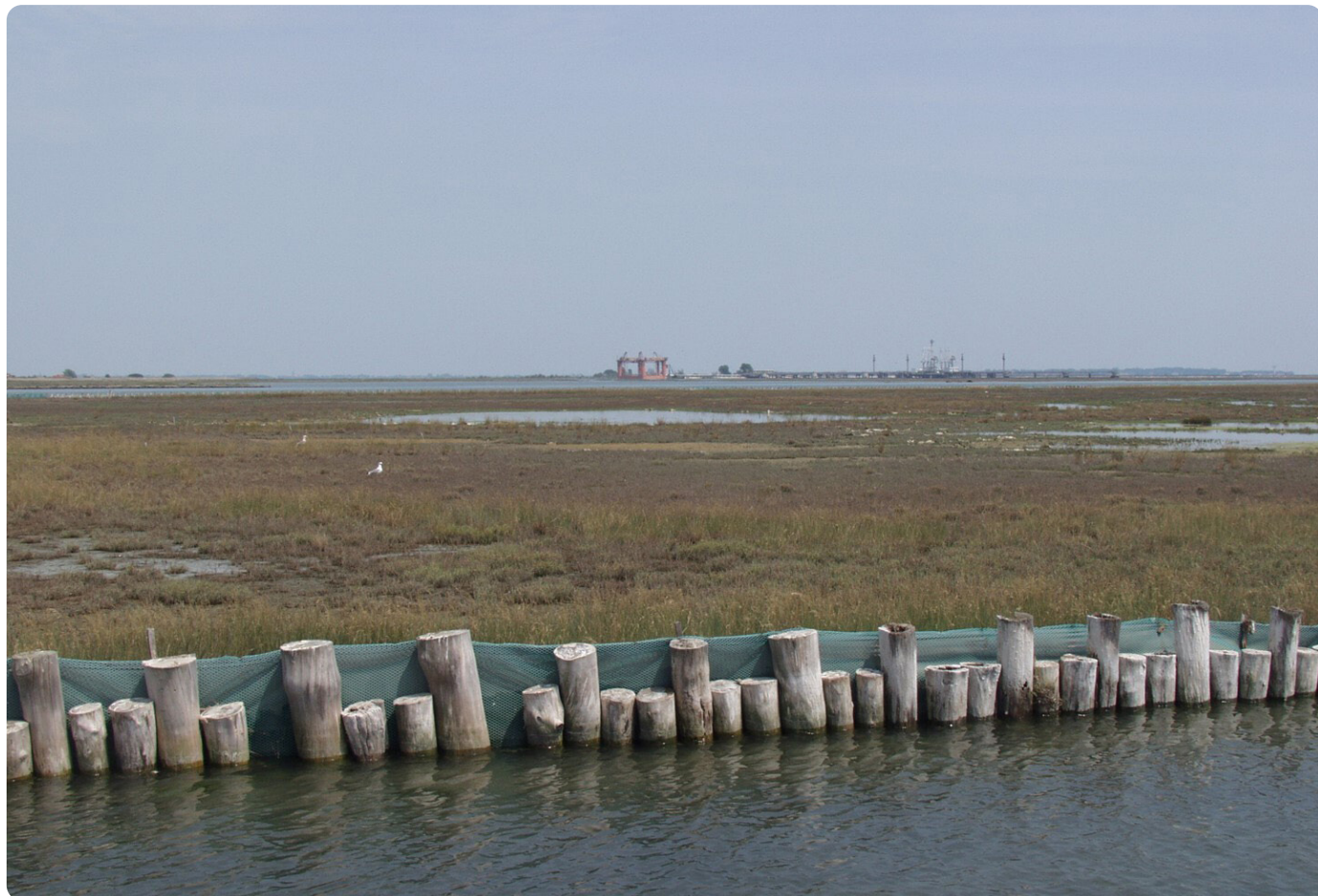
Piling technique to protect salt marsh edges
