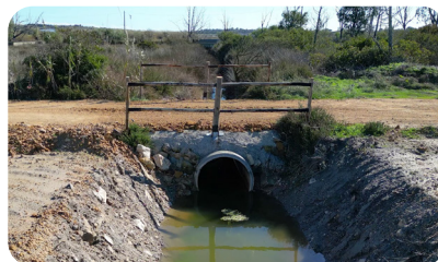
Connective channel dredging (between Cuba and Longarini)
