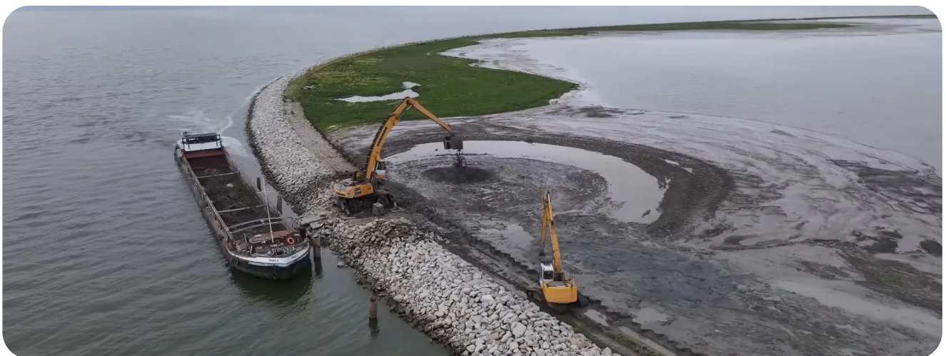
Ongoing restoration actions
