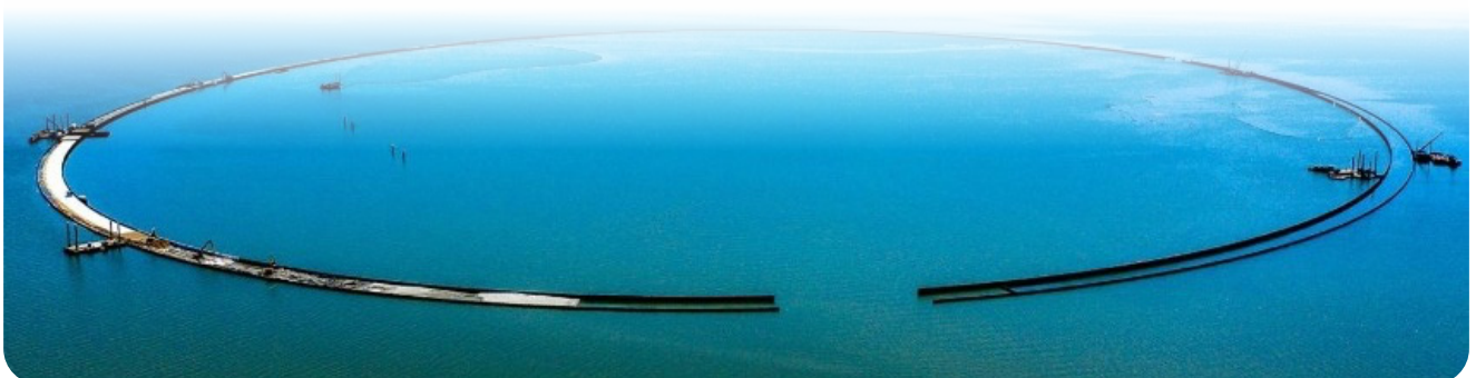
Area of future island ready for filling
