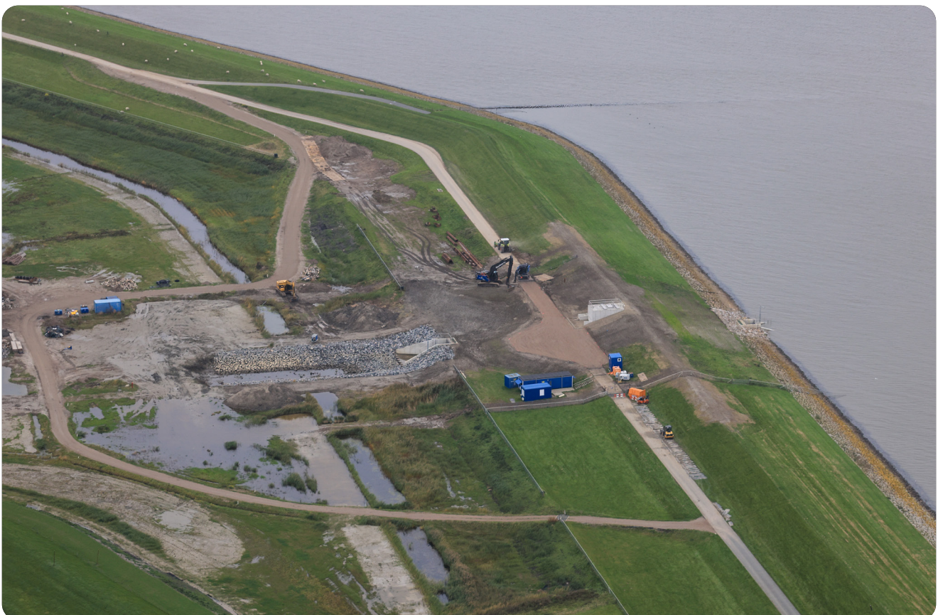
Construction of Double Dike
