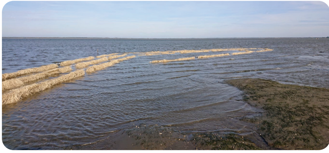
Artificial seagrass use to mitigate tidal current velocity in order to reverse the positive feedback processes to allow spontaneous recolonization
