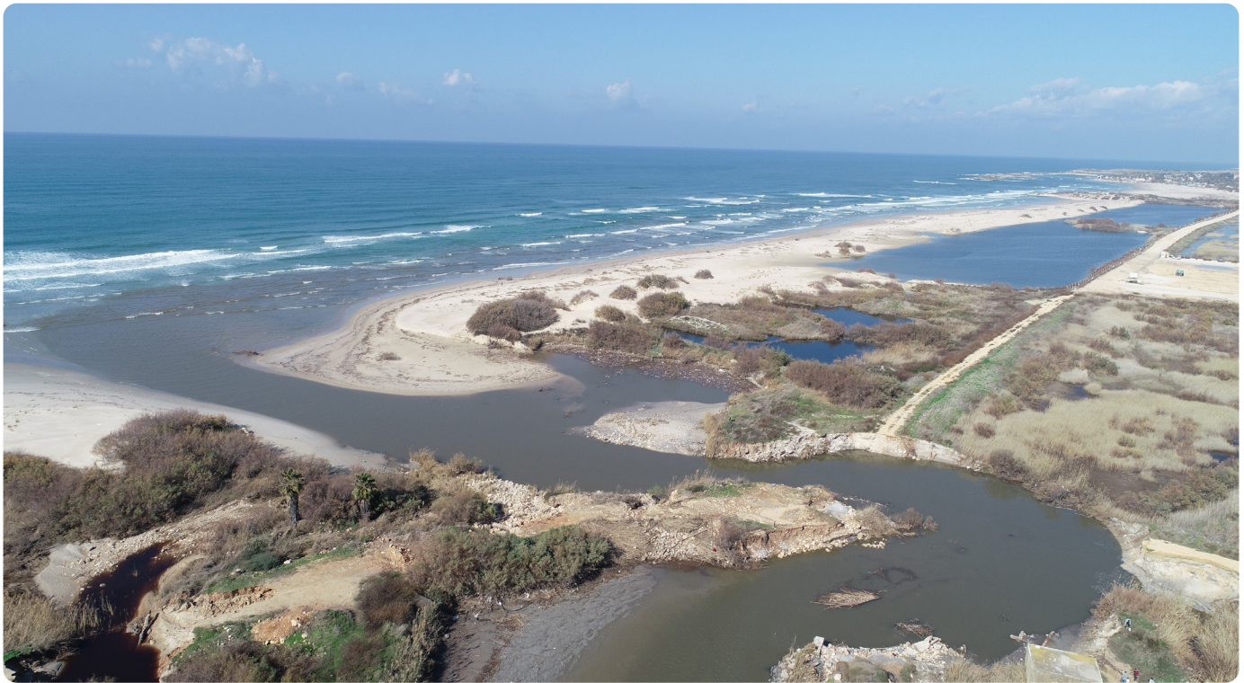
Earth-dam breaching during floods
