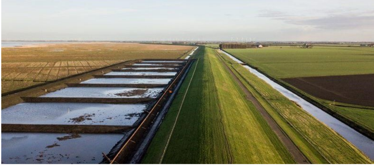
Figure 11: Project ‘Wide Green Dike’ ( www.eemsdollard2050.nl )
