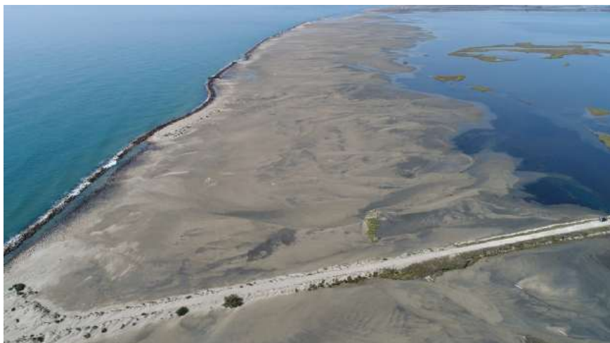
Figure 70 New beach area due to overwash process due to non-maintenance of outer dike (Willm & Béchet, 2023)
