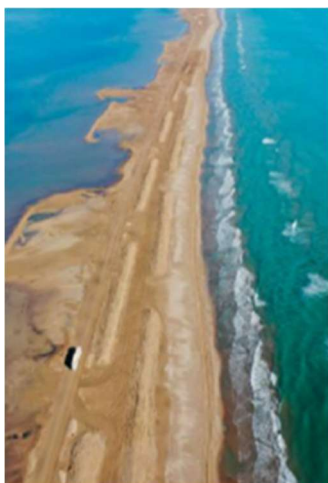
Figure 24 Drone image of the Trabucador barrier showing the system of alternating dunes (Eurecat & UPC, 2023)
