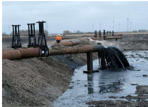
Figure 43 Depositing wet mud through pressure pipes during the pilot phase (ED2050, 2024)
