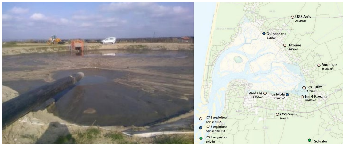
Figure 5.4. Sediment settling basin (left) and their location (right) [SIBA].
