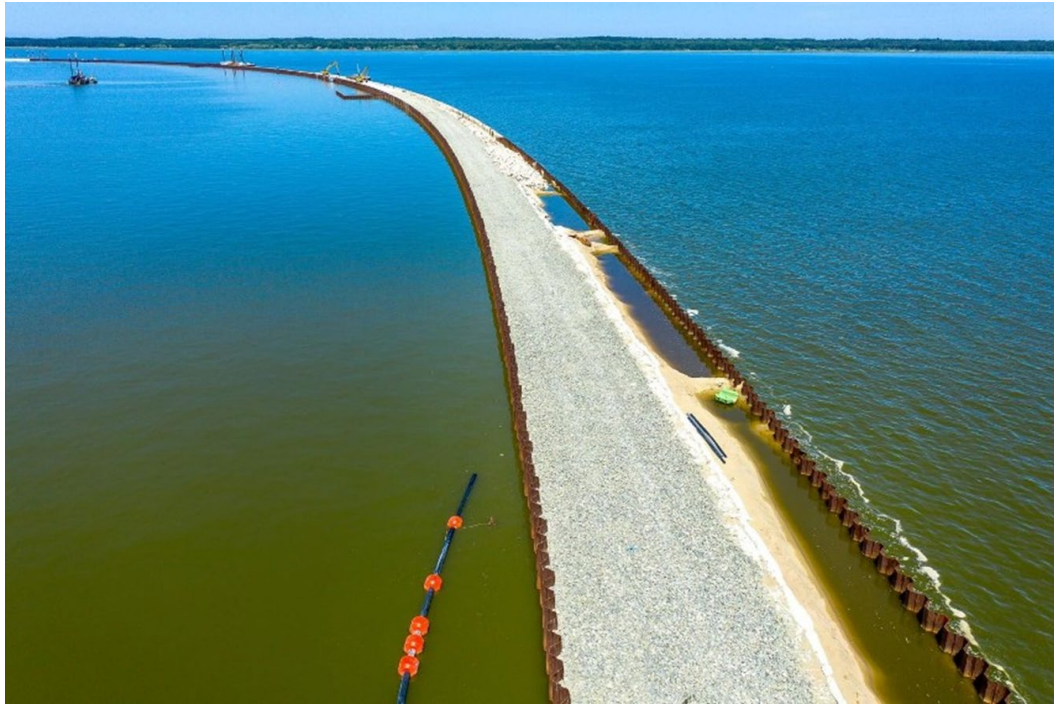
Figure 8.3. Rim under construction, made of two rows of sheet piles with stone armor gradually forming the crest between them: source - courtesy NDI group.
