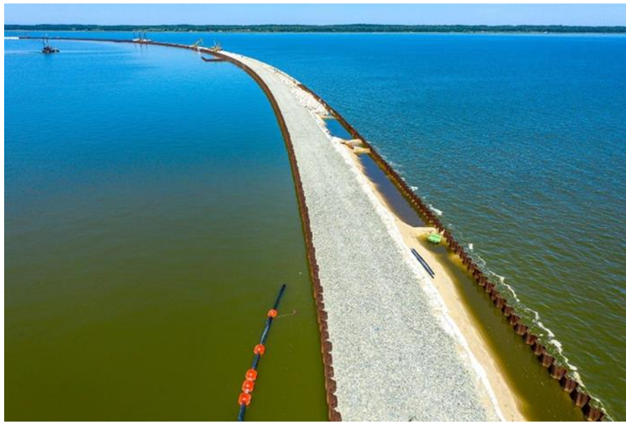
Figure 11-4 Low strength parameters of lagoon bed necessitated the rim made of two rows of sheet piles braced on top and filled with stones to resist ice phenomena
