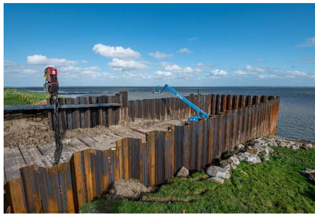
Figure 2. Inlet Double Dike under construction, as benchmark for Groote Polder.
