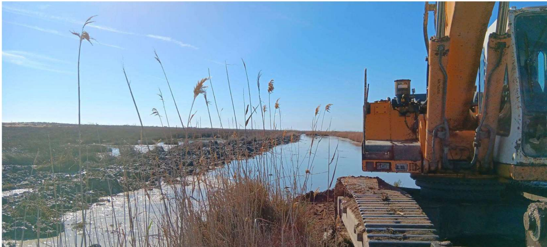
Figure 7. Restoration works in the Alfacada Lagoon consisting of the removal of the dike.
