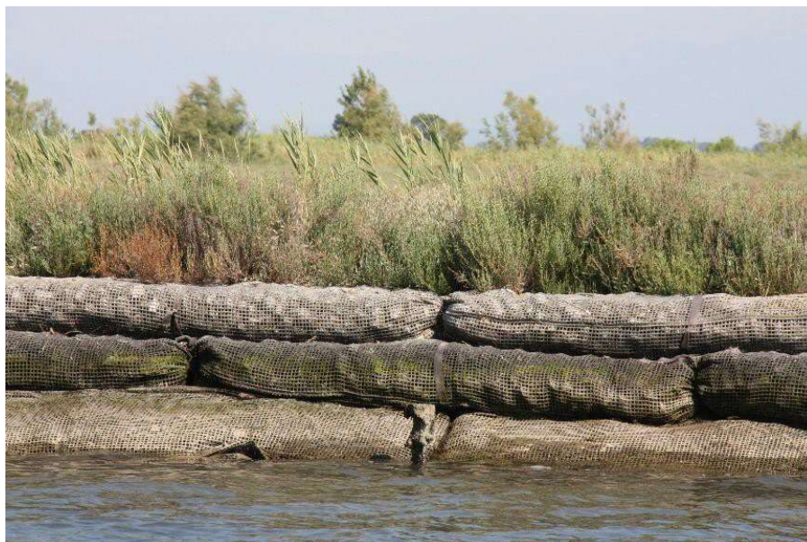
Figure 31: Example of a hybrid solution, with gabions on mattresses.
