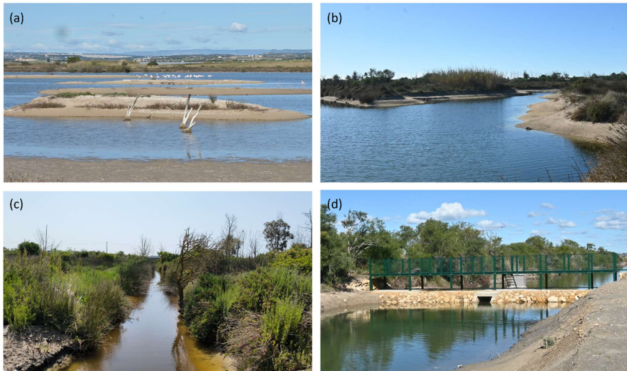
Figure 3: Ongoing restoration actions at Cuba-Longarini pilot site, artificial islands for bird nesting (a), coastal marshes restoration (b), restored channel between Cuba and Longarini lagoons (c), barrier and gate for lagoon water level regulation (d)
