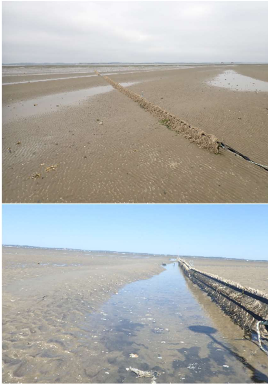
FIGURE 16. ILLUSTRATION OF THE DUNE / SCOURING PIT SETTLED AFTER ROSELIÈRE SOLUTION UNDER FLOW INFLUENCE
