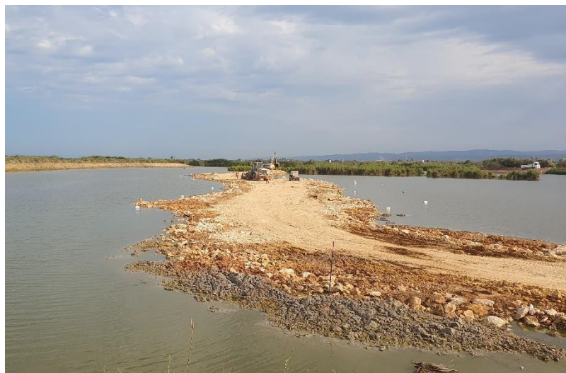
Figure 3: New battery that separates the water body on the northern reserve to two seasonal water bodies with changing water levels. INPA's project materials.
