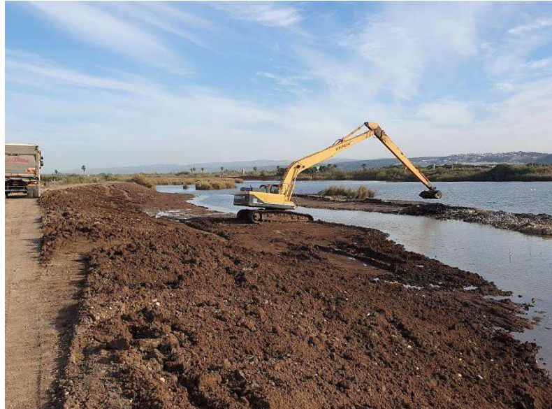
Figure 2: South-western bank restoration during works in the southern reserve. INPA's project materials.
