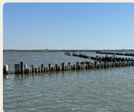
FIGURE 19. BEFORE-AND-AFTER RESTORATION AT THE VENICE LAGOON PILOT SITE. © ENG. GIOVANNI ASSALONE, DIRECTOR OF WORKS. PROVVEDITORATO INTERREGIONALE PER IL VENETO, TRENINO AA, FRIULI VENEZIA GIULIA
