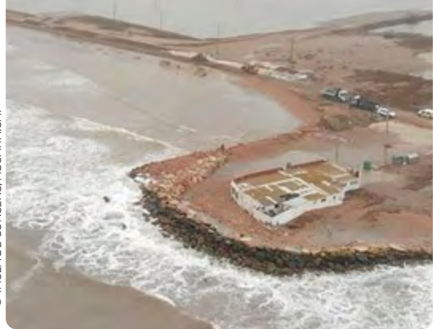
A rigid coastal defence structure protecting a historic restaurant from coastal erosion (La Punta del Fangar, Deltebre)
